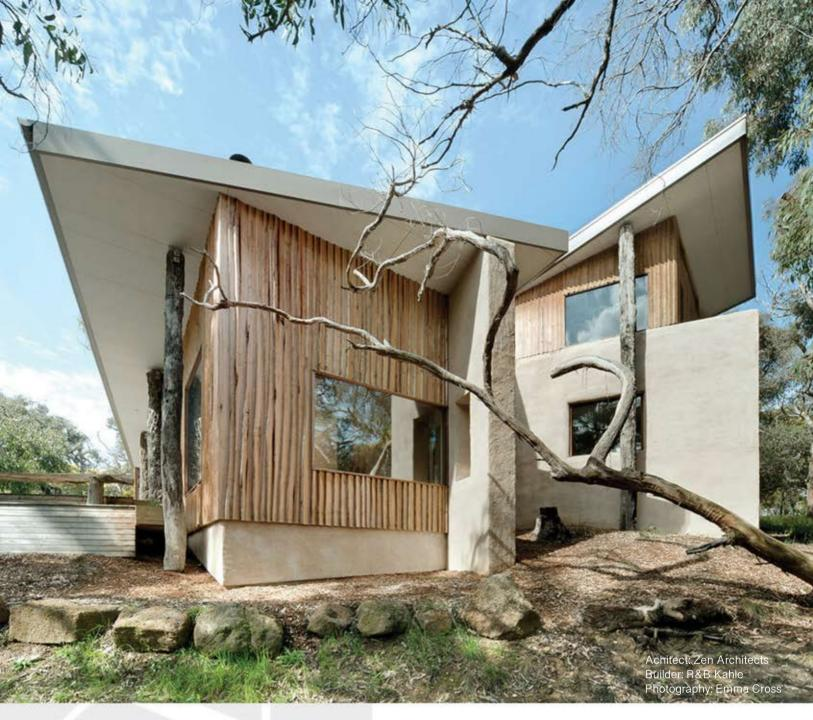
Radial Timber Natural Edge Weatherboards are a sustainable option providing a unique rustic barn style look which perfectly blends into the natural surroundings. Supplied unseasoned and transported to site in log form with the ends uncut, this radially sawn product is produced to provide stability with minimal waste. Natural Edge Weatherboards have been used as a feature on houses, commercial landscaping projects, visitor centres, communal playgrounds, holiday homes and sheds.
