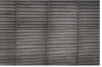
Logs come in a range of lengths from 3.0m - 5.4m so consideration of the length of wall is necessary. It's recommended that a 75x50mm sawn stop is used to break up longer runs into shorter sections or alternatively you can route a groove and lap join the boards.
