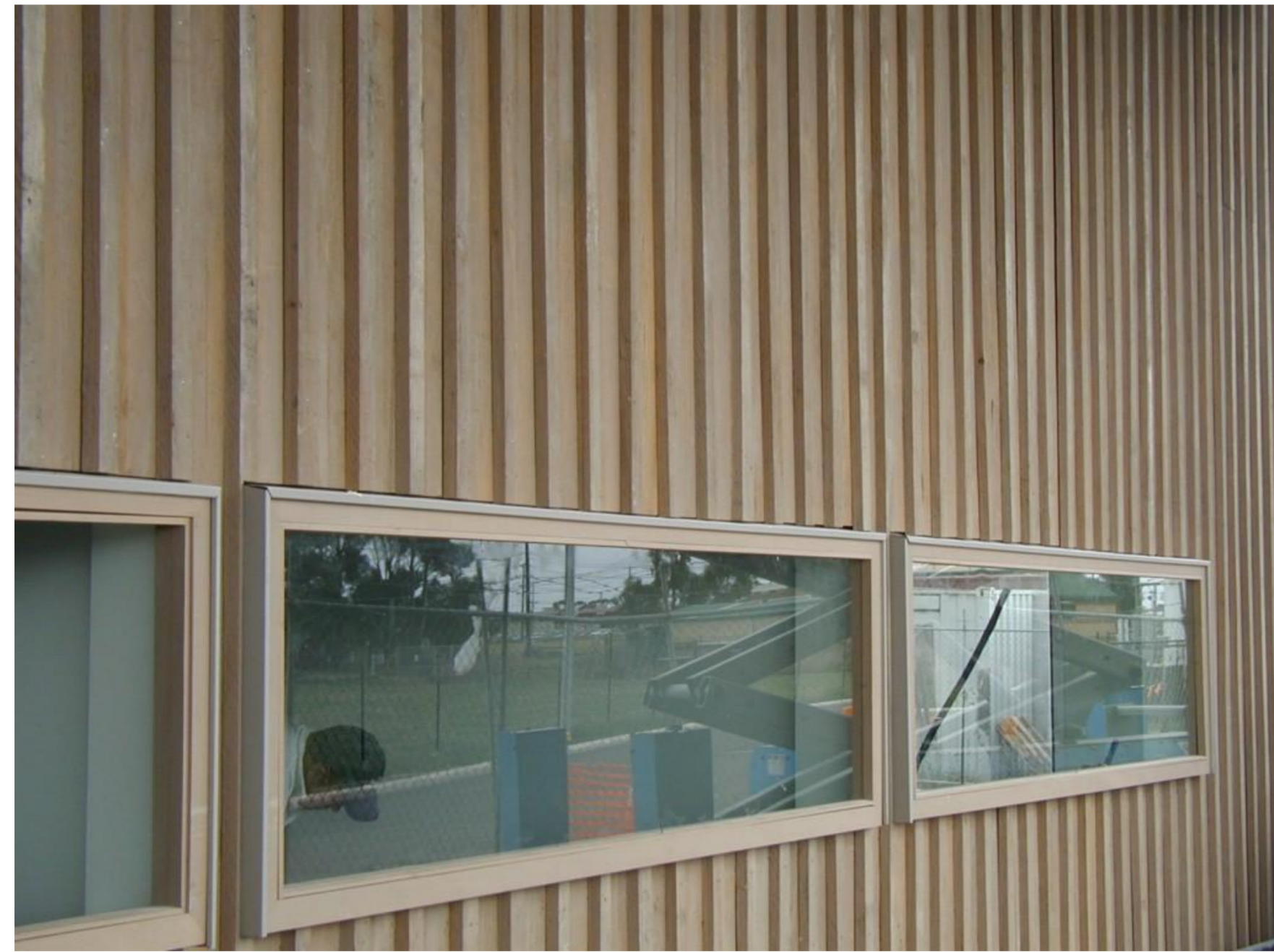
Typical Radial Bevelled Edge Board & Batten unseasoned rough sawn wall cladding with window/window flashing example inset
