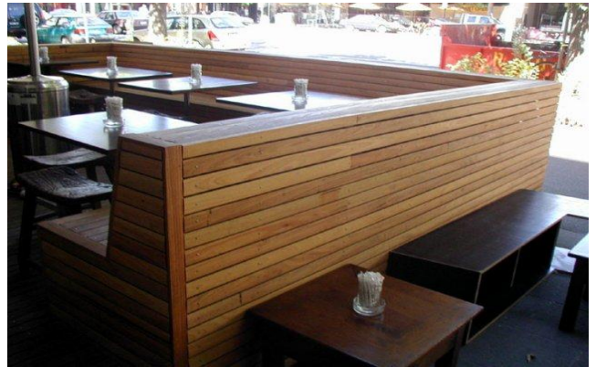
Yellow Stringybark decking(80 x 19) used for seating.
