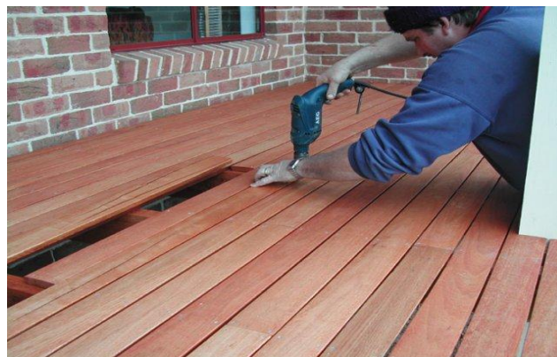
Installation of Southern Mahogany decking (100mm x 19mm)
